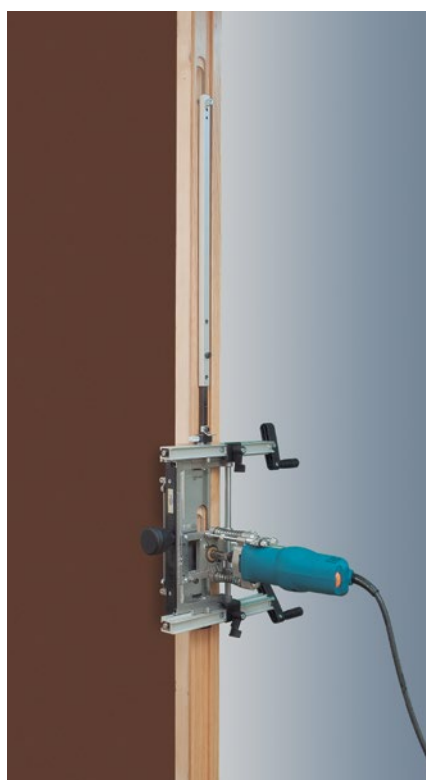
Making the second recess on the frame.
