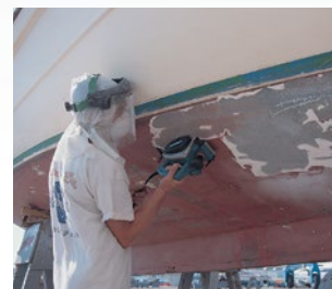
Maintenance work in shipyards.
