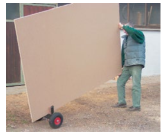
Carrying a large panel on an irregular floor.
